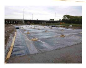
Currently, the first phase of the road construction is in execution. Pollux Consulting carries out the daily supervision of the bentonite liner placement
