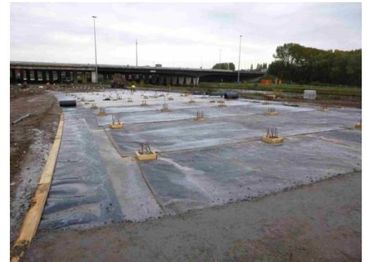
Currently, the first phase of the road construction is in execution. Pollux Consulting carries out the daily supervision of the bentonite liner placement
